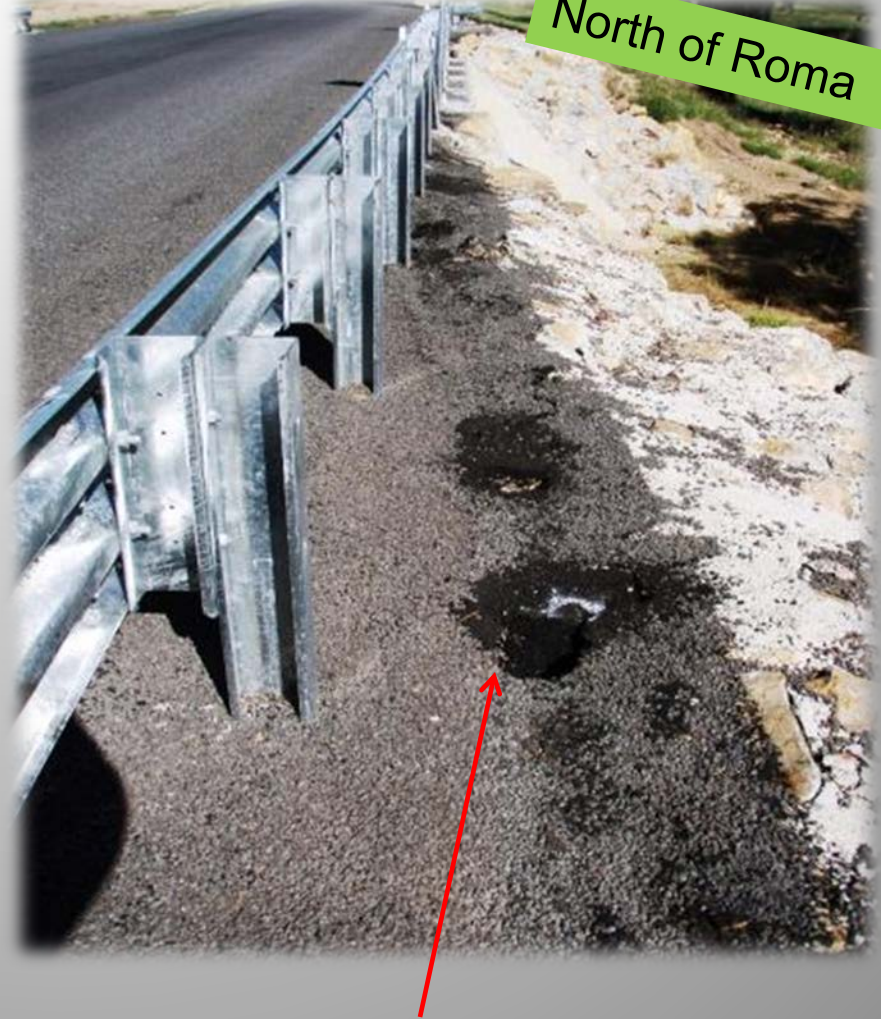
Erosion paths were grout injected
